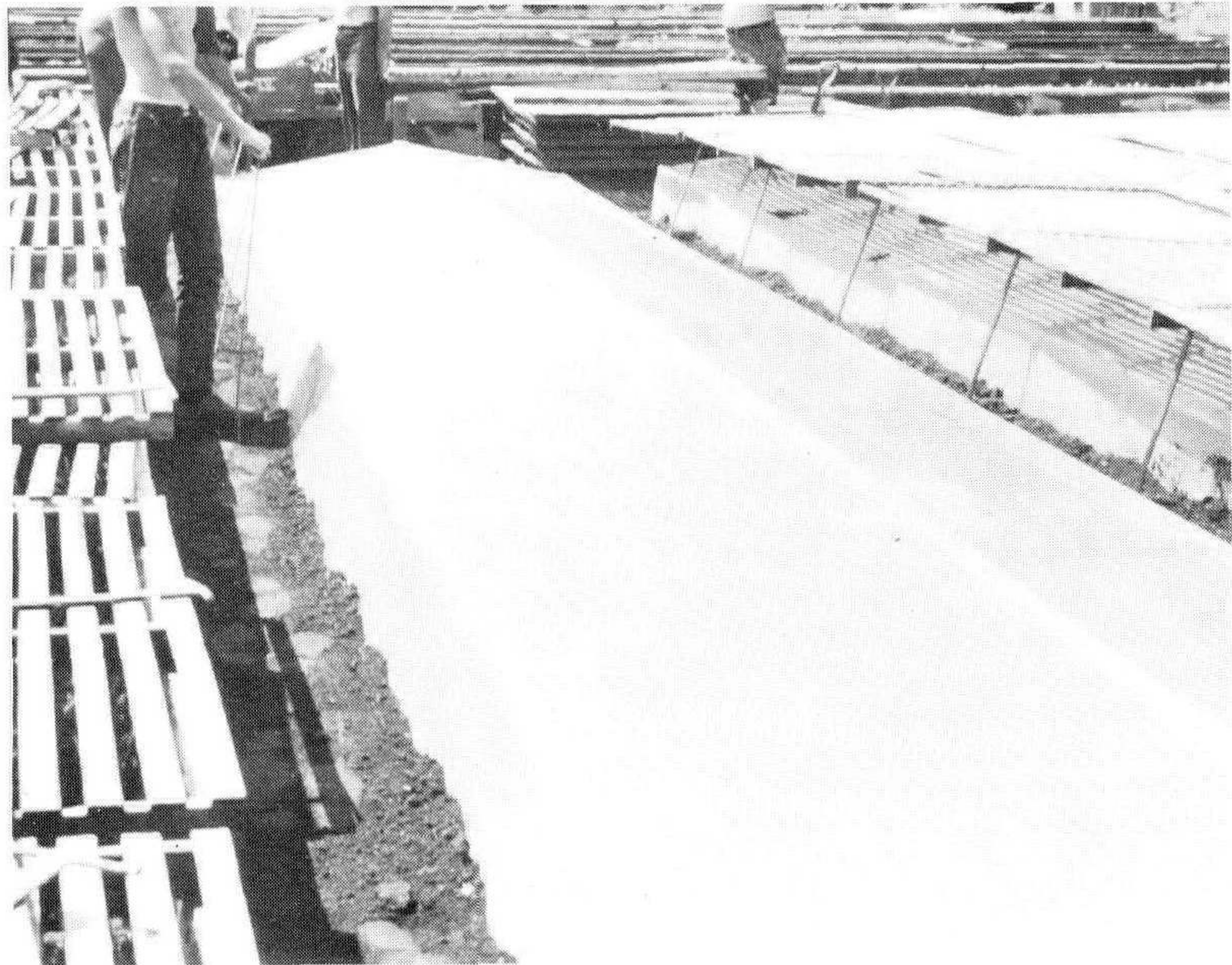
Fig. 2. Frame is covered with 4 mil polyethylene, soil is tamped along the sideboards and metal "T" stakes are set in place preparatory to covering it with lath shade.
