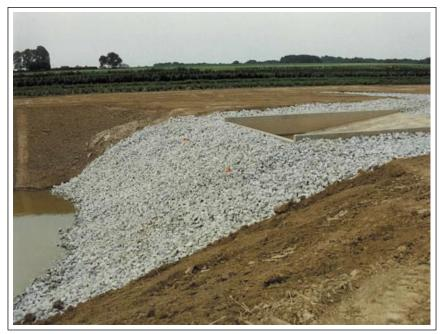
$\mathbf{Figure}~\mathbf{2.}~\mathbf{Rock}$  layer on the surface of the pond wall below the weir.
