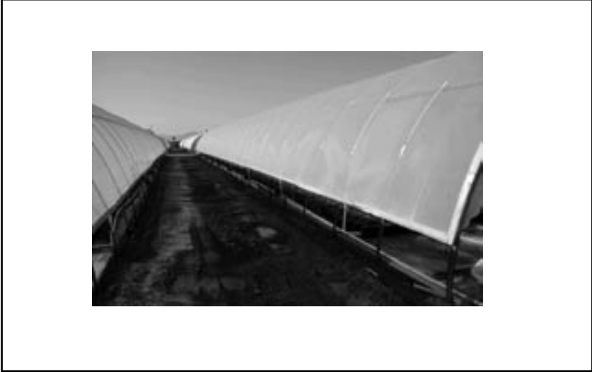
Figure 1. Quonset houses with side ventilation systems for better temperature control.
