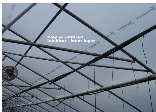
Figure 2. Polyethylene film with infrared layer to reduce heat loss.
