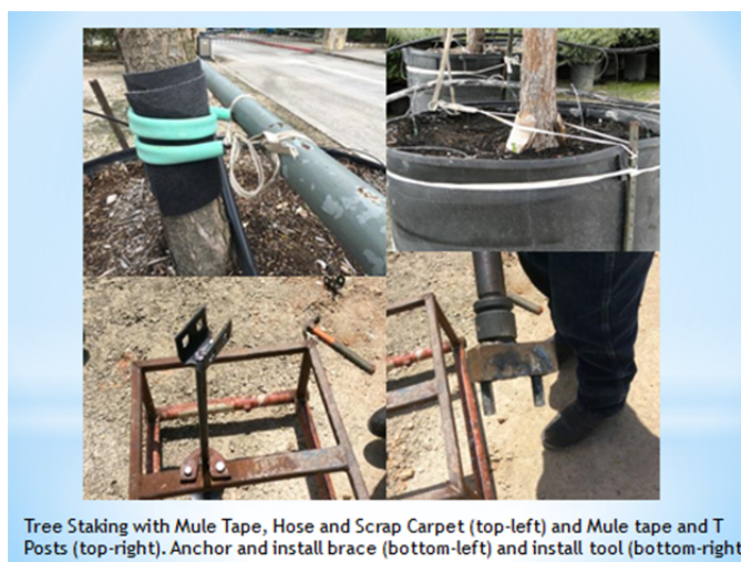
Figure 7. Tree staking with mule tape, hose, scrap carpet and mobile home anchors.
