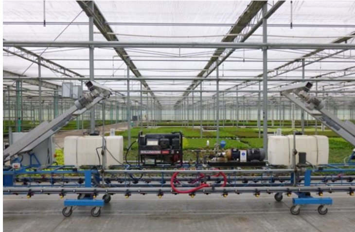
Figure 10. Automatic spraying machine using rail system.
