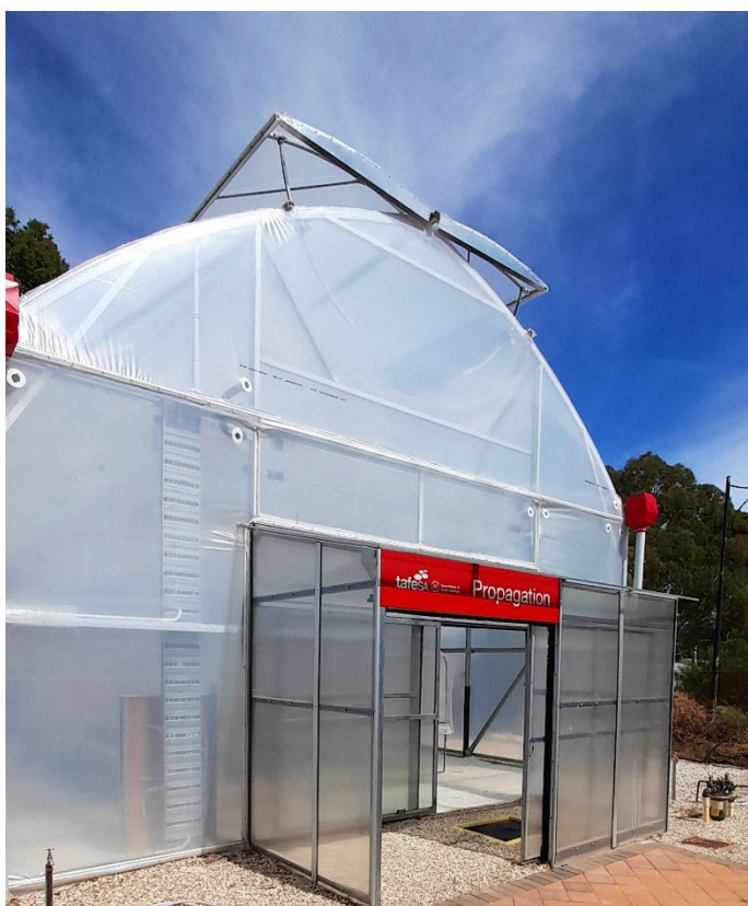
Top to bottom clockwise: The new facility features automated energy screens, an insect barrier and LED lighting to allow for night classes, climate control system supplied by Redpath, new facility from the front including hygiene vestibule and footbath.
